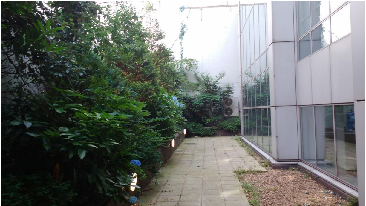
Courtyard area/ Ground floor level of office building
