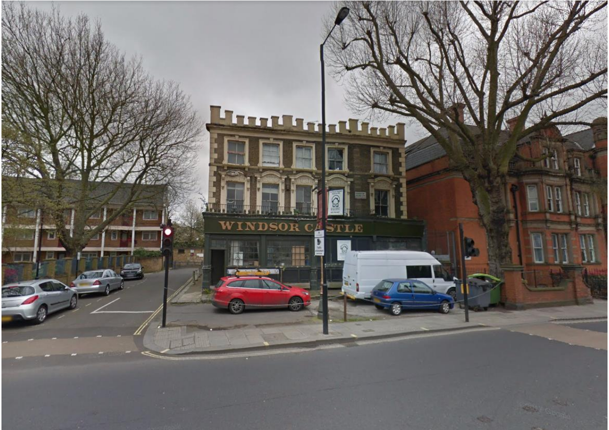
Frontage of application site as seen from Harrow Road and Chippenham Road intersection.
