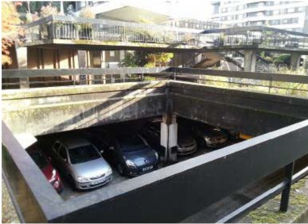
Example of Existing Lightwell
