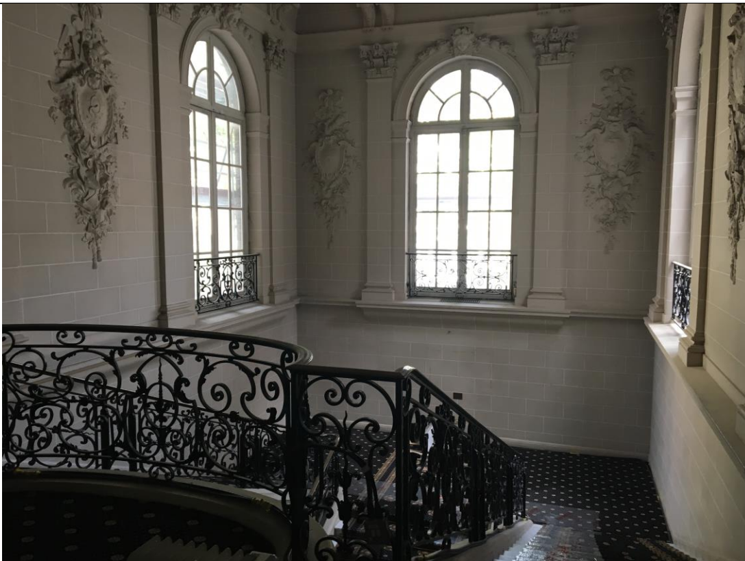
Main Staircase from First Floor
