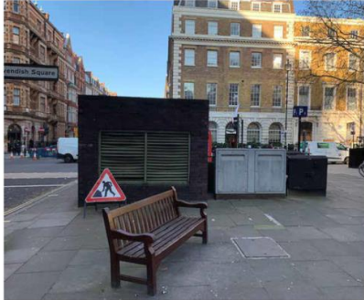
3M HIGH PLANT ENCLOSURE & STAIR- NORTH-EAST CORNER
