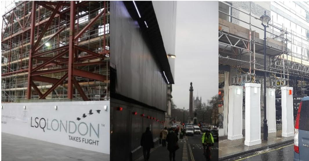
*Temporary luminaires mounted on building support frame and poor practice where the existing column-based lighting is included within the scaffolding*
