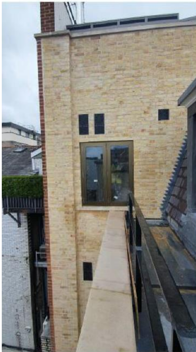
Rear lightwell facade
