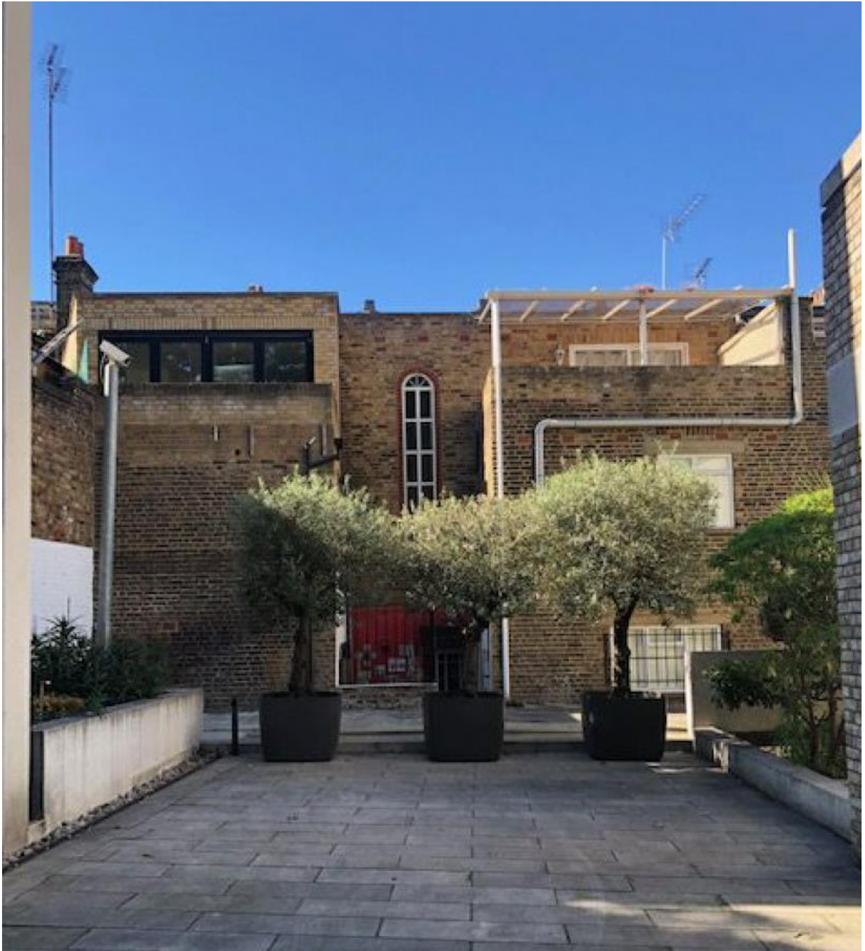
Rear Elevations of nos. 11 (left) and 10 (right).
