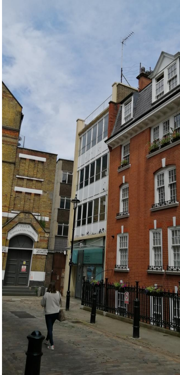
Front elevation from the junction of Foubert's Place and Marshall Street
