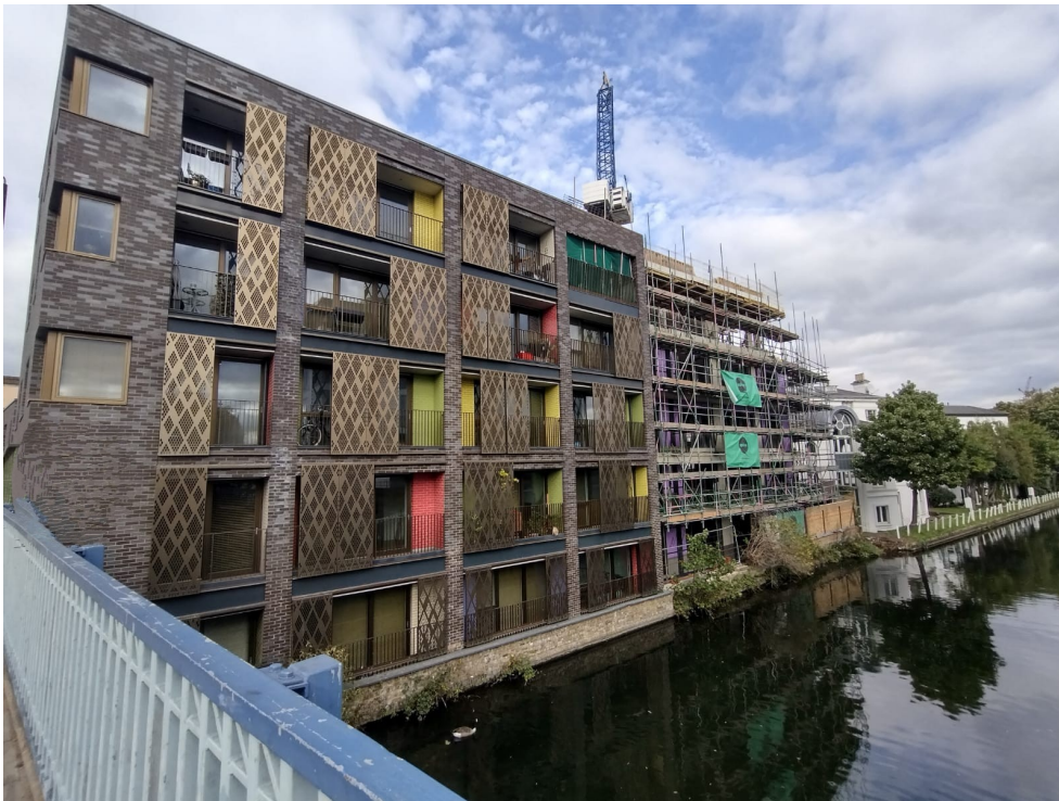
External rear elevation of Victoria Wharf Phase 1 and Phase 2
