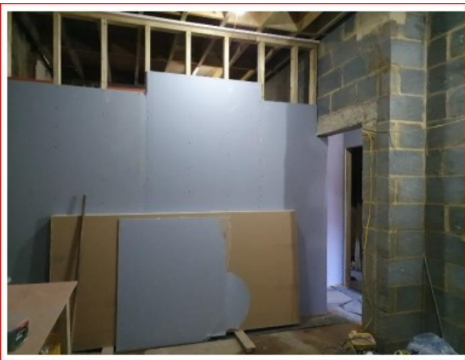
Ground floor partitions
