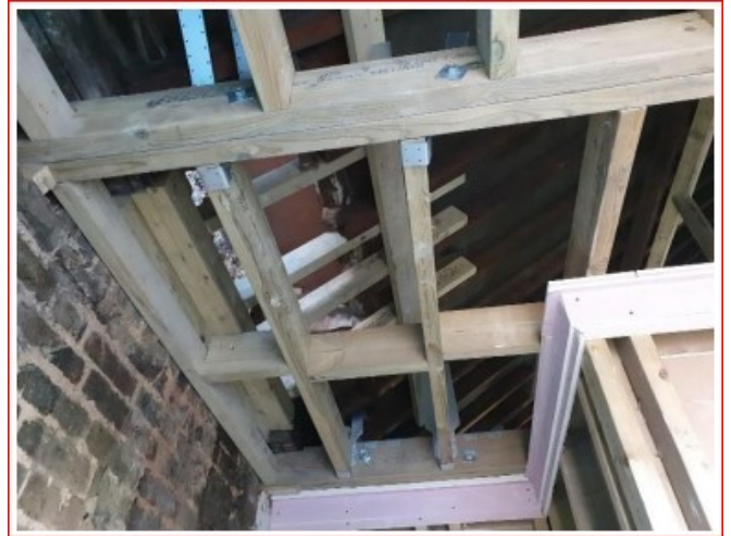
Roof rafter chimney repair
