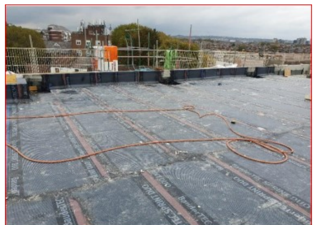
Water proofing on main roof
