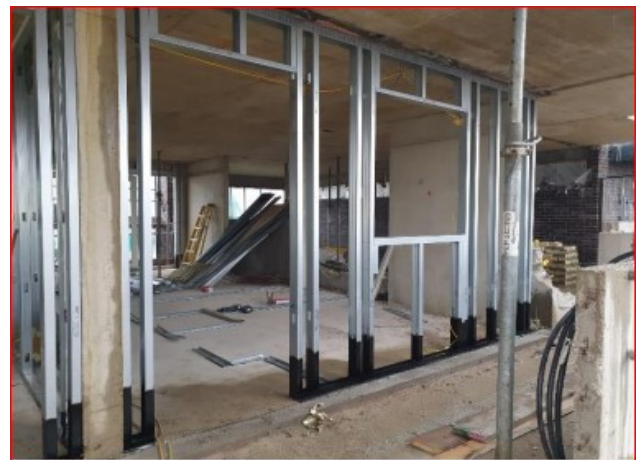
Third floor partitioning
