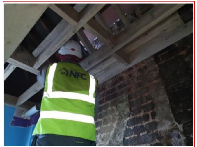
Second floor ceiling joisting
