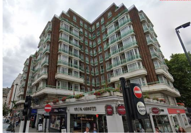
View of corner of Melcombe Place and Gloucester Place.
