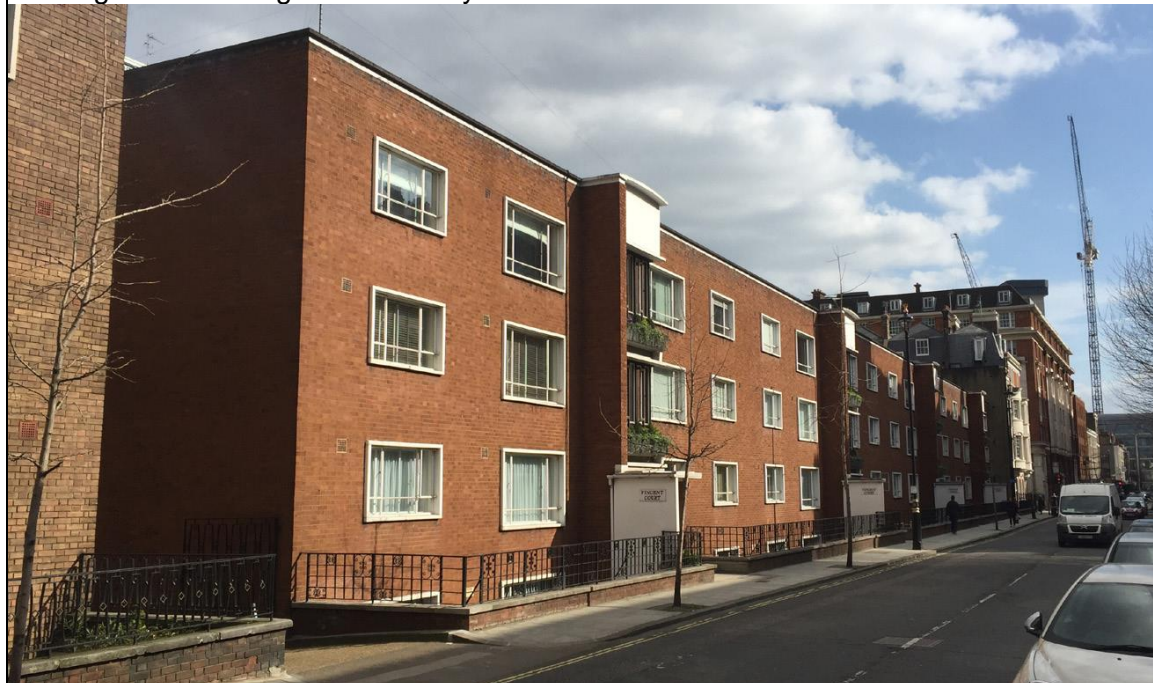
Existing View Looking South on Seymour Place
