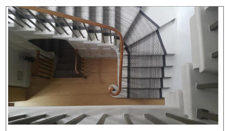
**Photograph 1** – view from first floor landing of the ground floor base of the staircase, showing also the existing (modern) stub stair flight down to the lower ground floor that would be removed.
